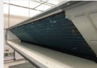
EPS foam drain pan with ABS resin coating
